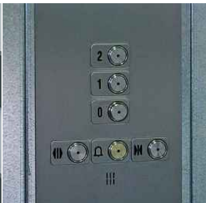
Car control panel of stainless steel, vandal-proof
